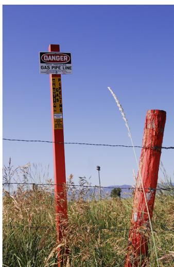
Pipeline markers show the approximate location of pipelines and identify the companies that operate the pipeline. Pipeline markers, sometimes called right-of-way markers, are placed at frequent intervals along transmission and distribution pipeline right-of-ways, public road crossings, railroad crossings, and other prominent points along the route.
