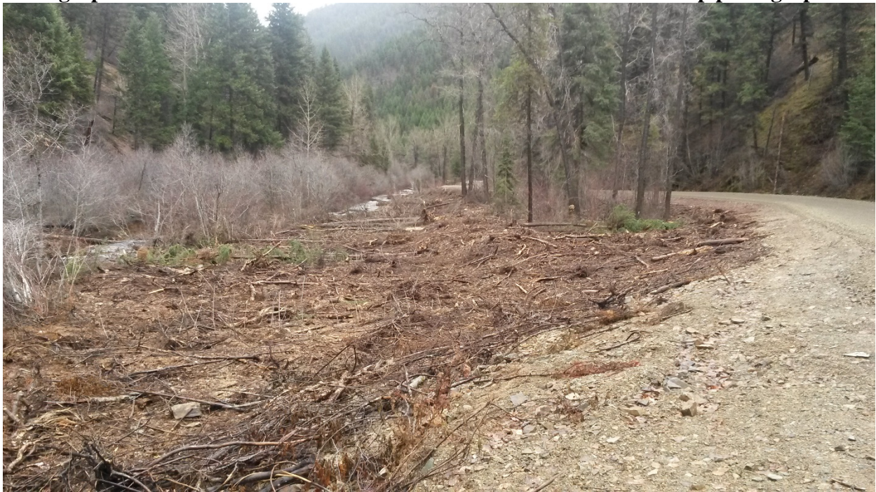
Photograph 4: Post construction. Picture taken from behind vehicle in top photograph.
