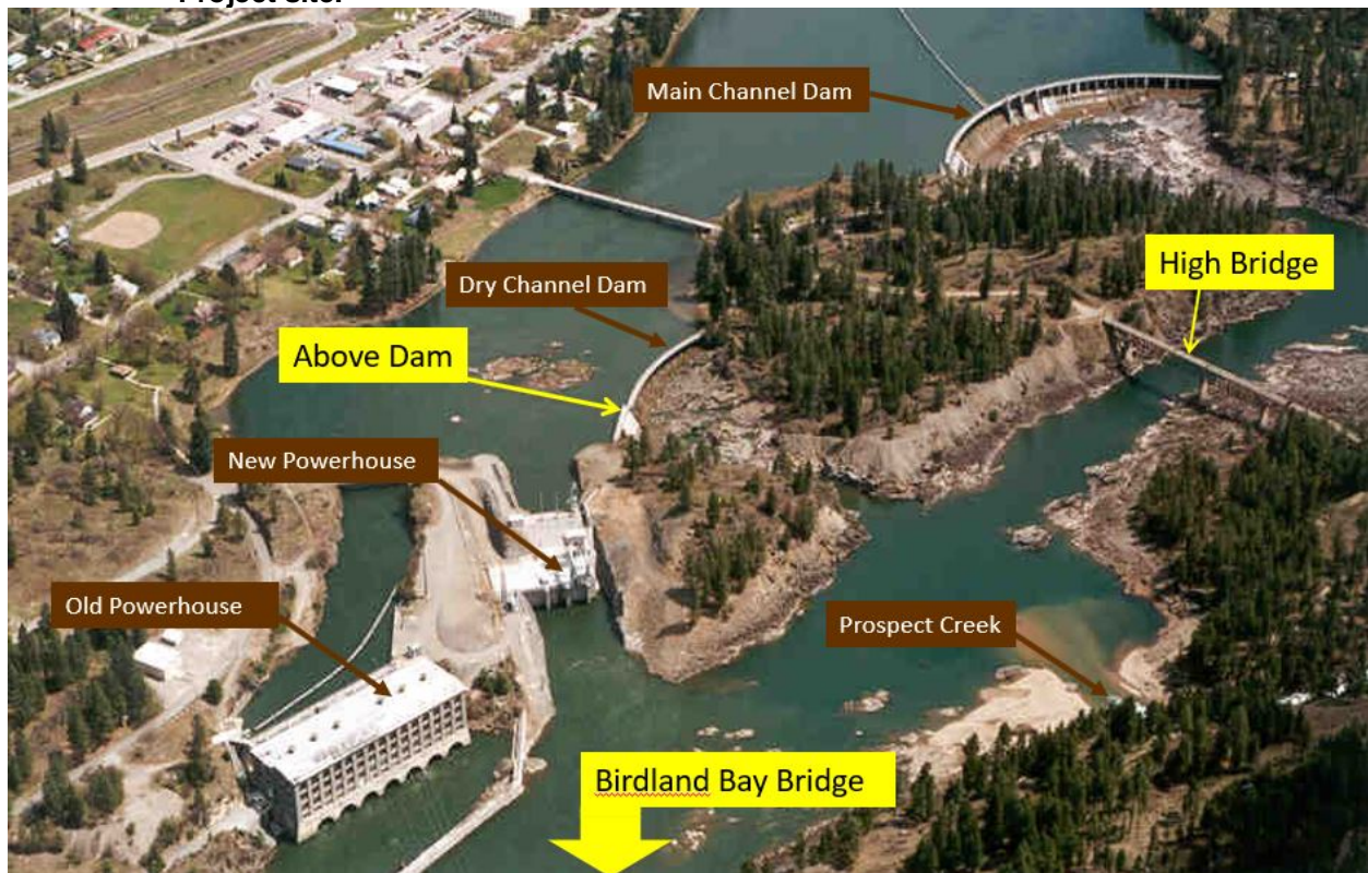
Figure 7-1: Monitoring locations for total dissolved gas at the Thompson Falls Hydroelectric Project site.
