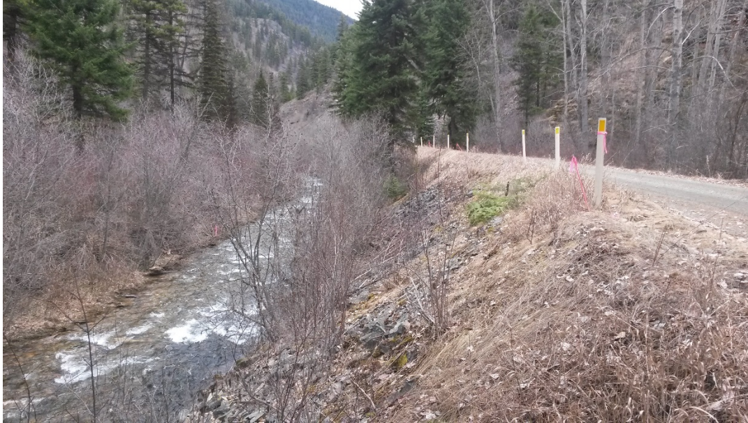
Photograph 5: Before and after road relocation. Note floodplain creation for high flows, canopy cover development and sediment filtering.
