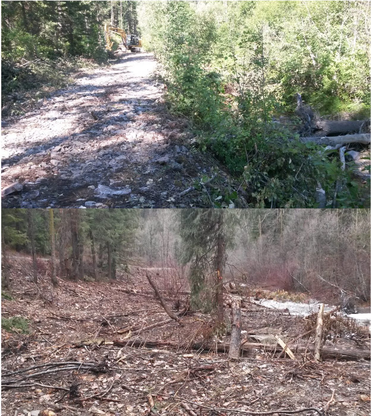
Photograph 2: Before and after removal of historic waste rock used for road construction and mining.
