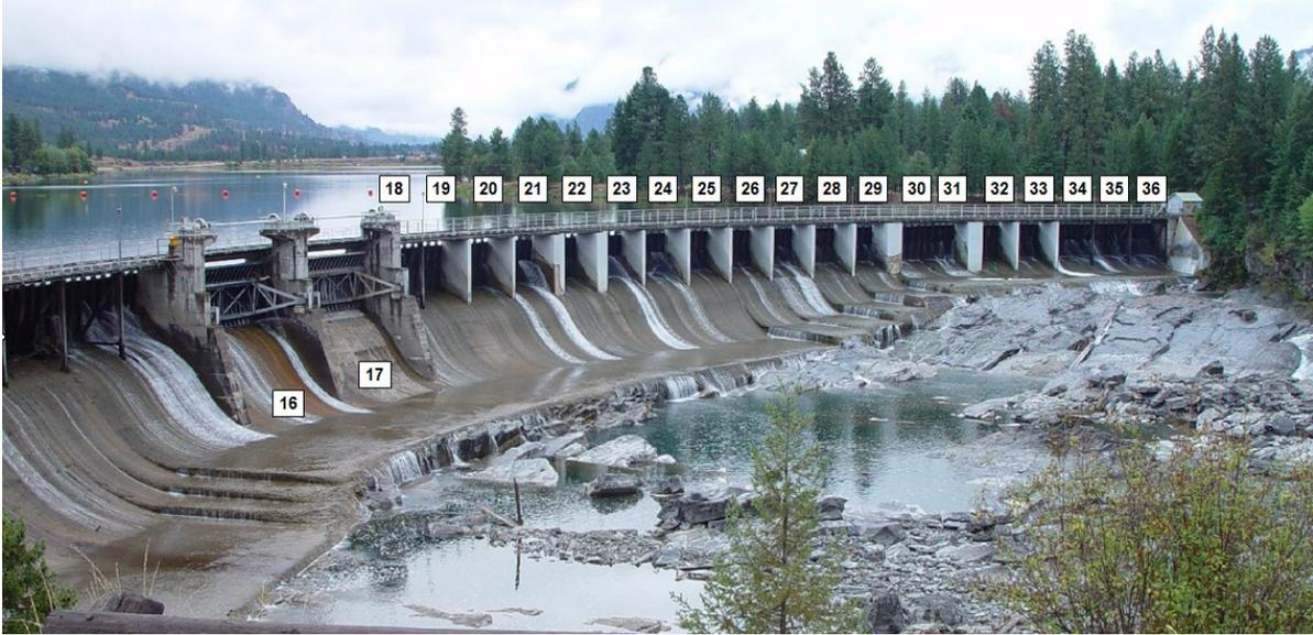
Figure 6-5: Operational Plan for the Main Dam Spillway applied in 2011.
