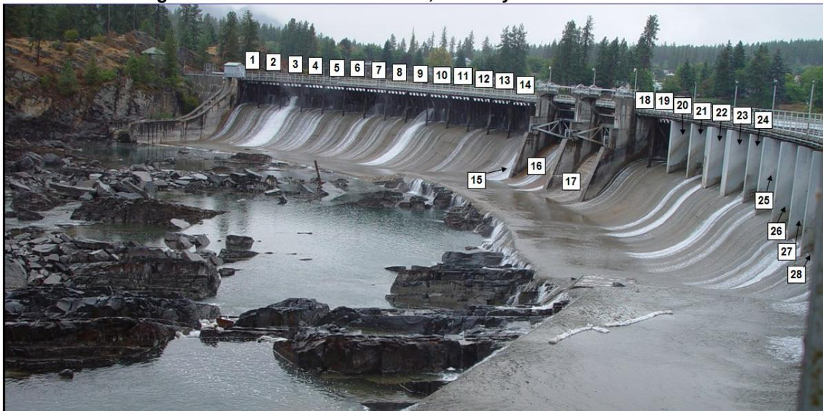
**Photo 6-2: The left bank of the Main Dam at the Thompson Falls Project, with the spillway bays numbered.**
