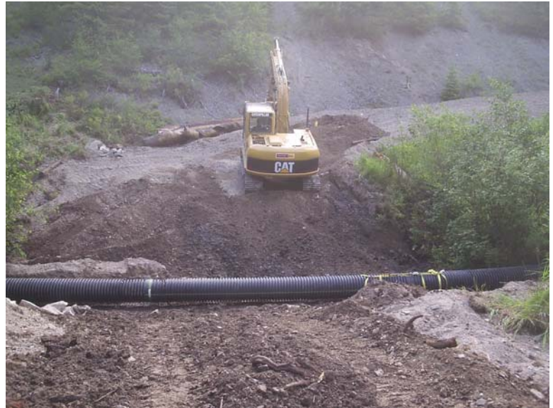
Dewatering at Wig Creek culvert removal
