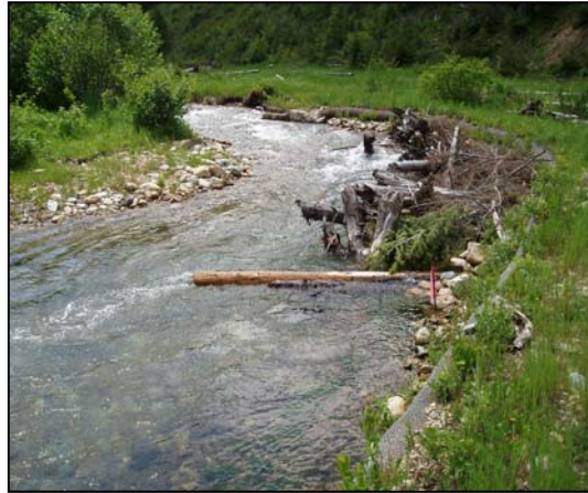
Figure 2-11. A vegetated soil lift and constructed ELJ following spring runoff and at the start of the growing season.
