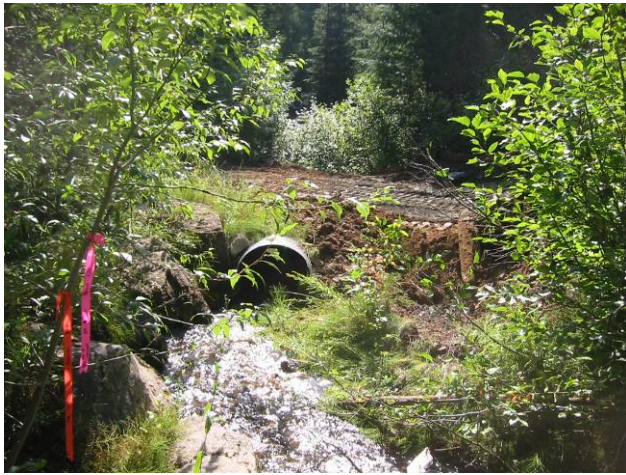
Surveyor Creek's lower culvert being prepped for removal.
