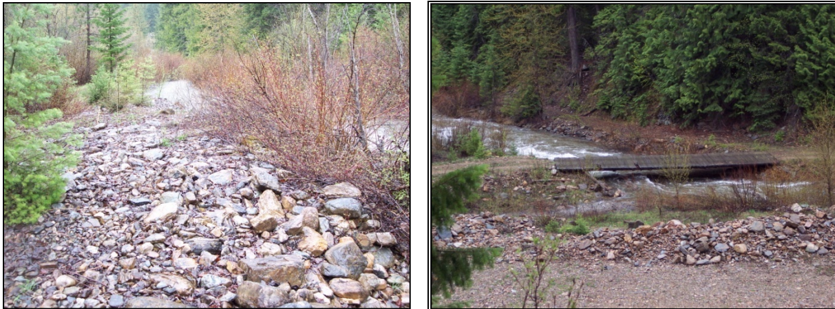
Figure 2-2. Oregon Gulch has been channelized in Reach 1 of the project area. Floodplain berms and the existing bridge constrict the channel and confine the belt width of Oregon Gulch, altering hydraulics and channel-floodplain connectivity.
