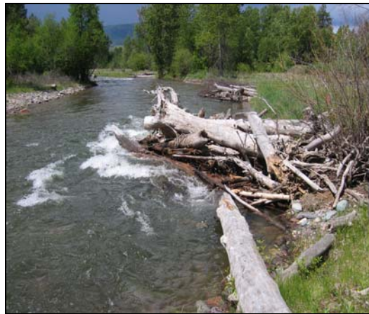
Figure 2-10. An ELJ constructed on the Jocko River in western Montana following two run-off events.
