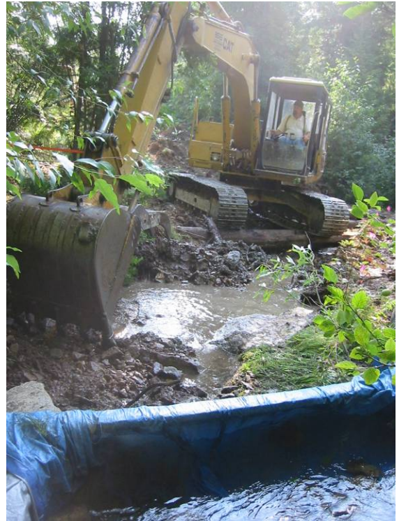
Rebuilding the stream channel with an excavator (and with hand labor).
