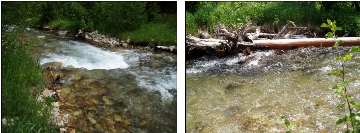
Figure 2-9. Example habitat improvement structures including low stage log and rock step-pools (left photo) and self-ballasted large wood aggregates.
