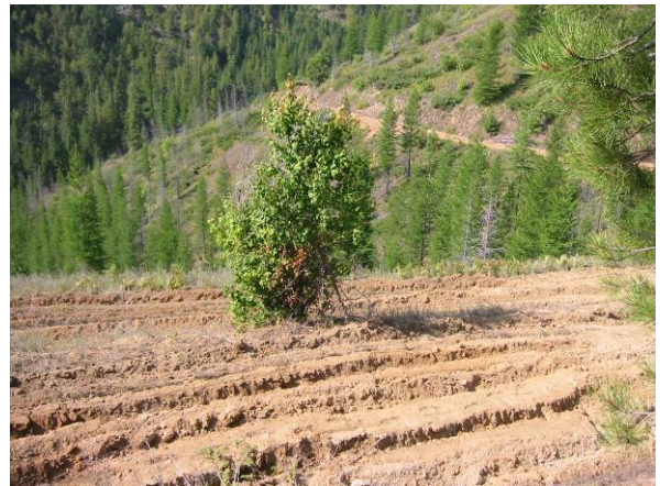
Over 40 miles of roads in Fish Creek have been decommissioned under this grant: weeds sprayed, surface ripped to 18 inches, culverts removed, cross-drainage added, and reseeded.
