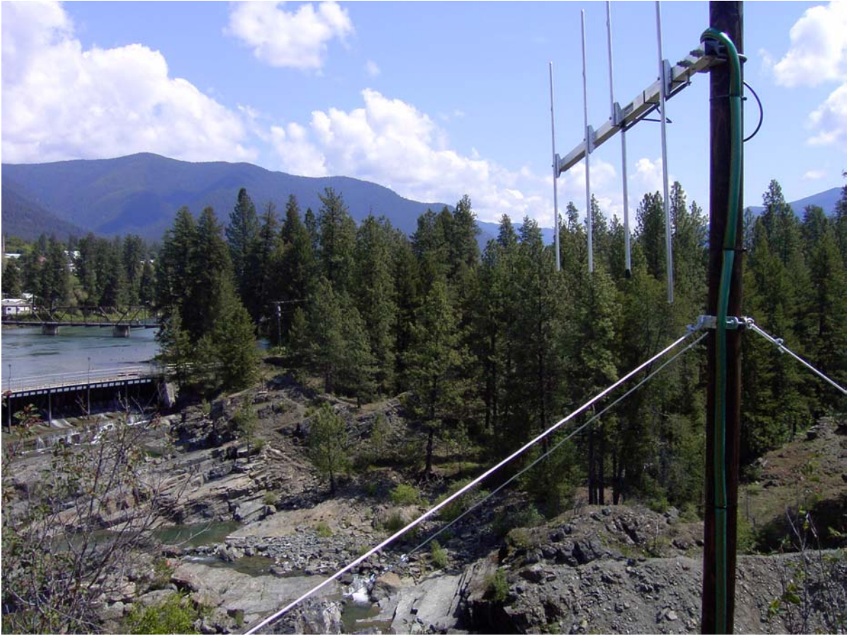
Photo 6. Antenna A of Hilltop telemetry station. Antenna A encompasses the area behind the dry channel dam.
