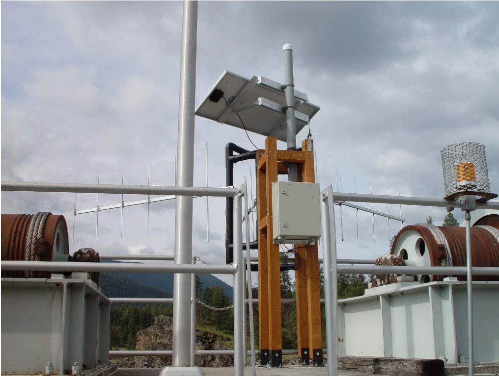
Photo 7. Main channel dam telemetry station. Antenna 3 is directed towards the right and encompasses the right side of the area behind the main channel dam. Antenna A is directed towards the left and encompasses the left side of the area behind the main channel dam. Antenna 0 is directed between Antenna's A and 3 encompassing the Clark Fork River downstream of main channel dam.
