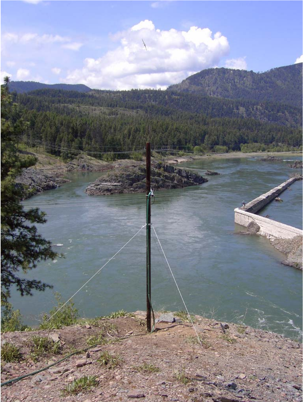
Photo 3. Antenna 4 of the Hilltop telemetry station, it encompasses both the entrance to the new powerhouse tailrace and the mainstem Clark Fork River downstream of the island.
