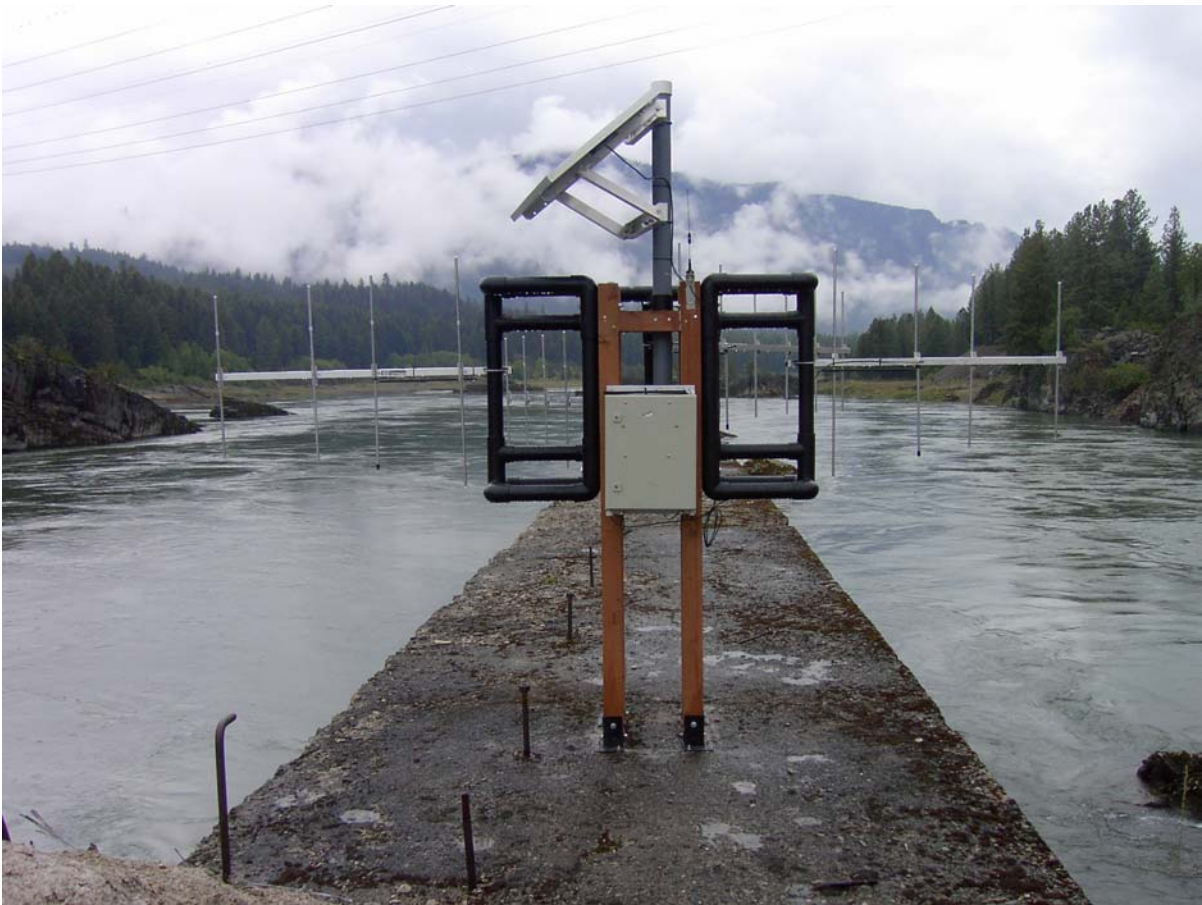
Photo 2. Wingwall telemetry station showing antennas. Antenna 5 is directed to the right and encompasses the tailrace of old powerhouse, Antenna 1 is directed right at an approximate 45° angle encompassing the entrance to the wingwall channel, Antenna A is facing left at a 45° angle encompassing the mainstem Clark Fork River downstream of the wingwall, Antenna 6 is facing left at a 90° angle and encompasses the mainstem Clark Fork River directly adjacent to the wingwall. Antenna 7 is not shown; it is positioned on the right bank facing into the new powerhouse tailrace.
