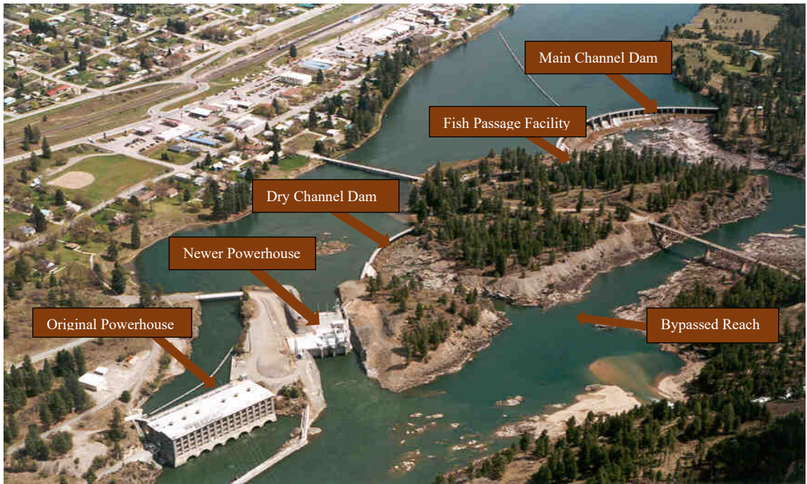
Figure 2: Major Project Features for the Thompson Falls Project (Source: PAD; staff)
