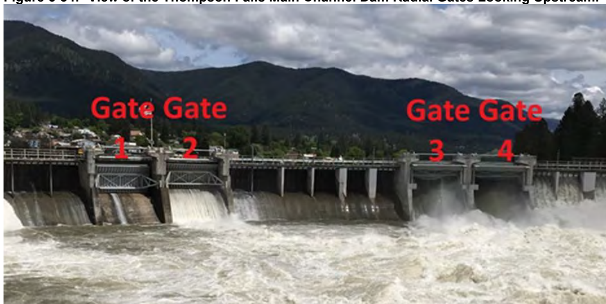
Figure 6-34: View of the Thompson Falls Main Channel Dam Radial Gates Looking Upstream.
