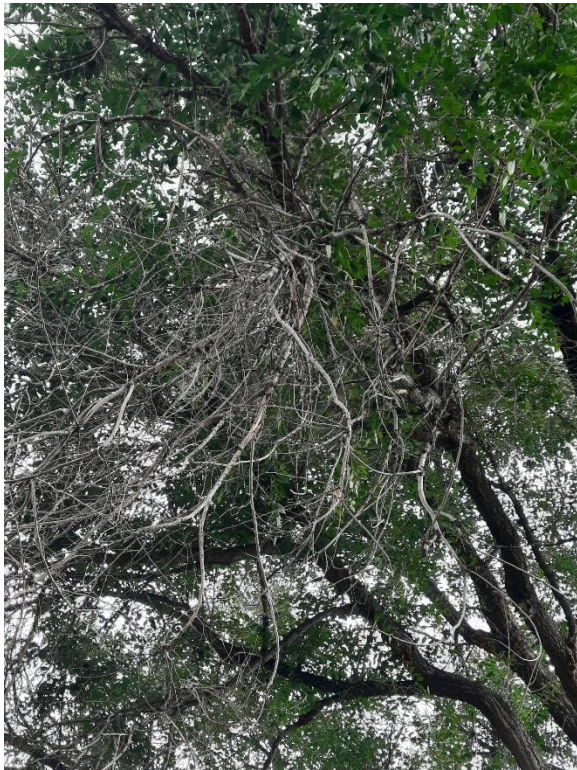
Hazardous tree branches in Headwaters picnic ground
