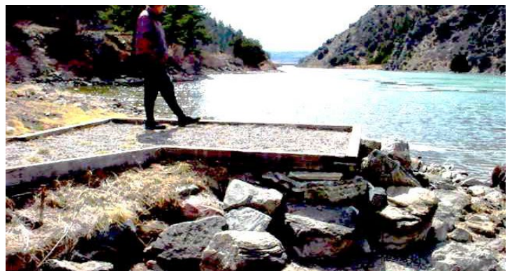
12. Original Photograph: rock fishing platform pre-stabilization
