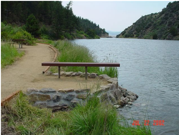
13. Original ADA route with fishing platform (post-stabilization)
