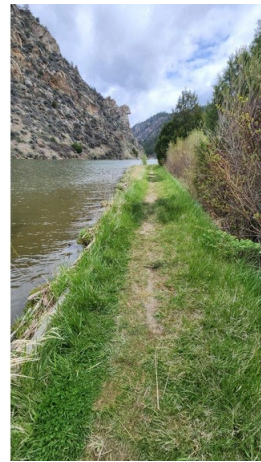
4. Former ADA route heading downstream, overgrown
