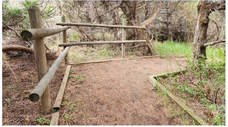
2. Current ADA route section at corner
