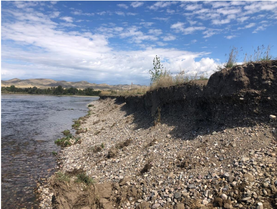
Figure 4. Photo showing the sloughing, unstable banks looking downstream from the confluence.
