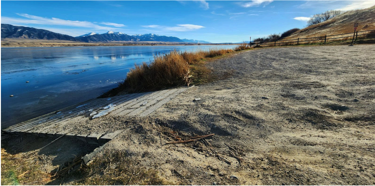
Attachment 3: Clute's Landing Boat Ramp – Erosion, Rutting
