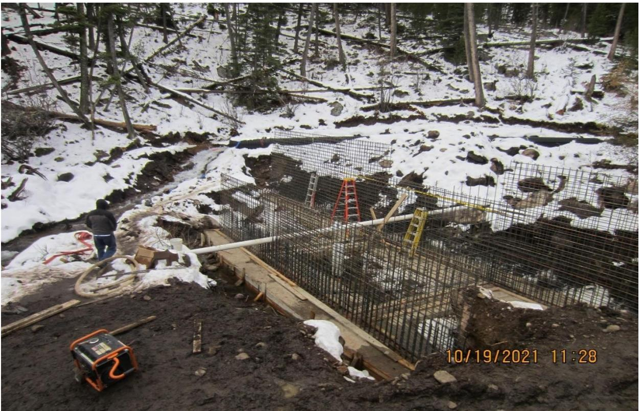
Figure 17. Wall Creek concrete barrier forms.
