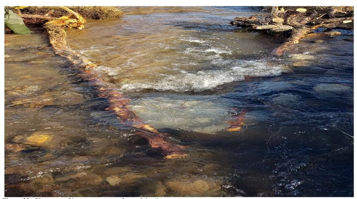
Figure 23.- Placement of instream structure for pool development.
