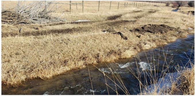
Figure 22. -Berm material removed to reconnect flood plain.
