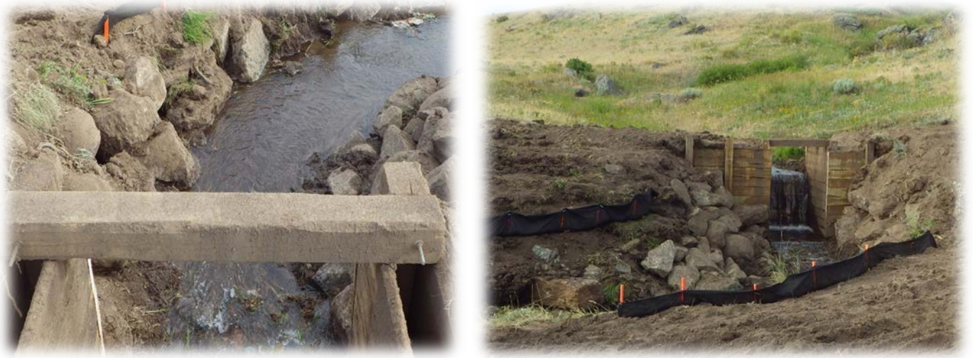
Figures 28. English George barrier installed view from top looking downstream and view looking upstream at the drop created.
