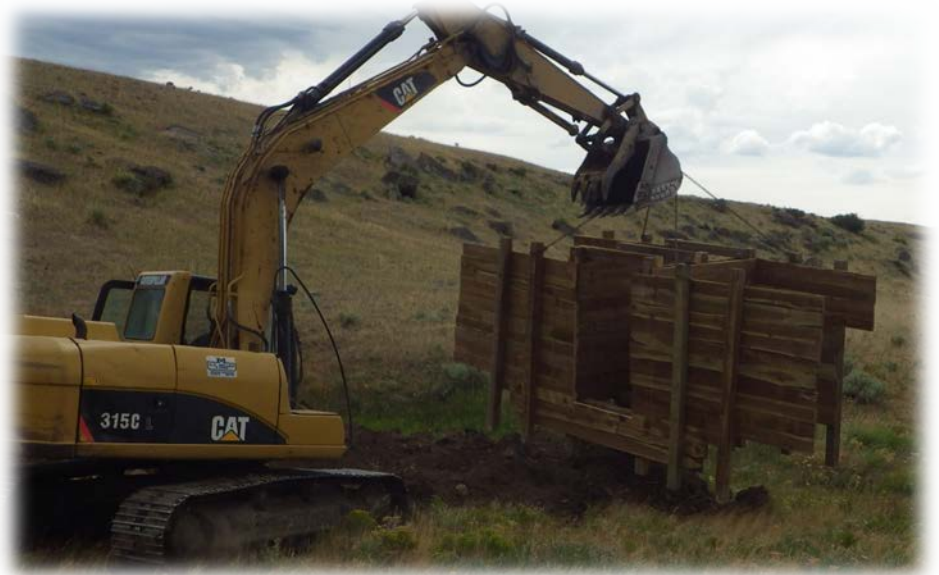
Figure 26. English George barrier being brought to installation site and being staged for placement.
