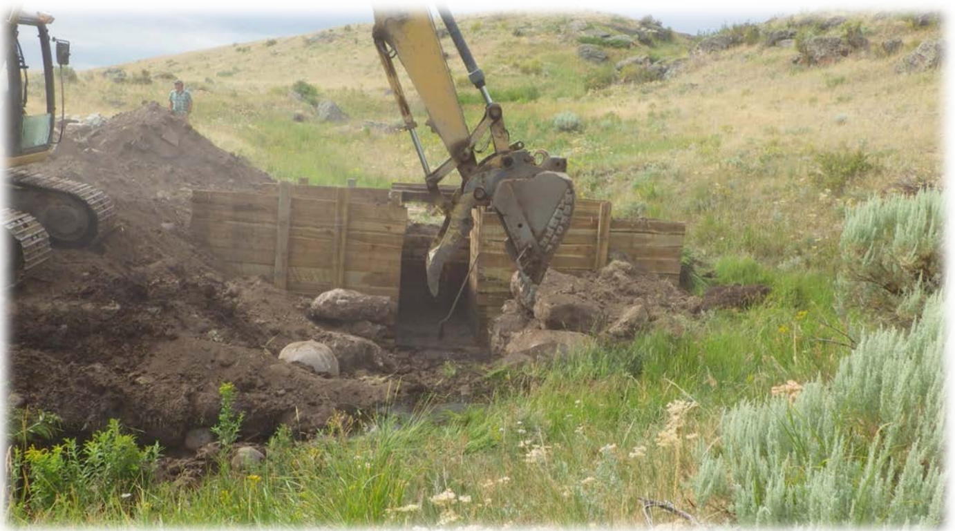
Figure 27. English George barrier in place and stream channel being fortified on the downstream side of the barrier.
